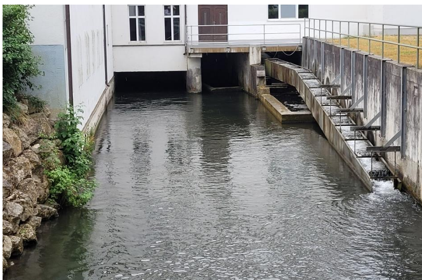
Figure 17: Outputs of the water from the small hydropower plant visited and its fish pass (La Jeunesse, June 2023)
