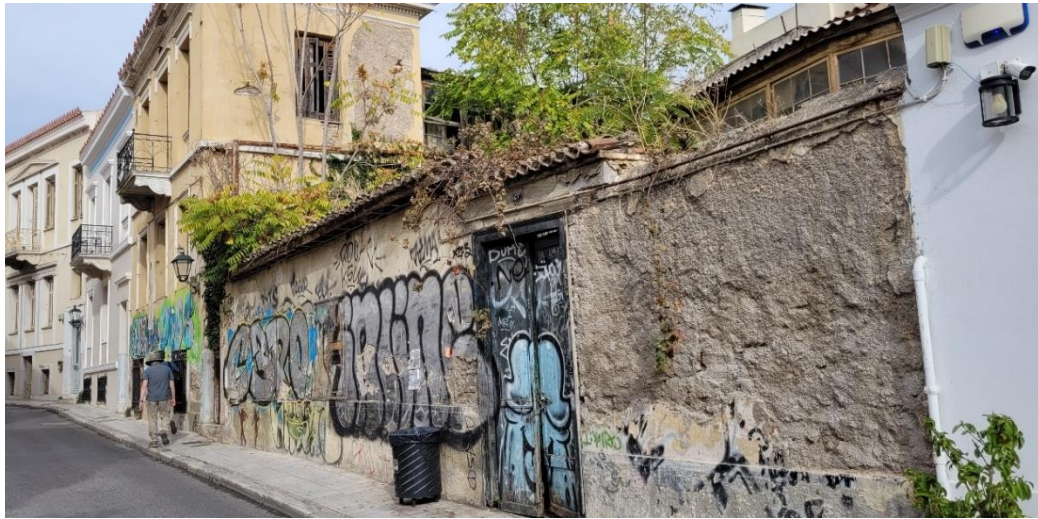
Figure 10: Example of derelict houses in the historic centre of Athens
